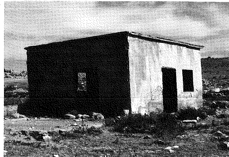
Figure 33. Building 1 in the JIV.
